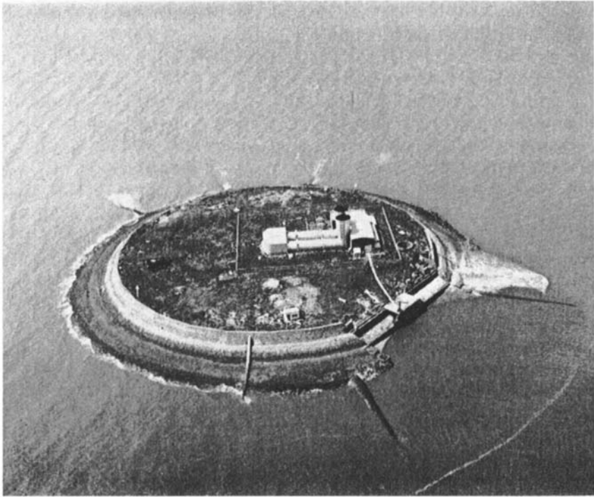
Figure 8.9 Hatsu-shima, an artificial island containing air ventilation systems for Mitsui's undersea collieries
