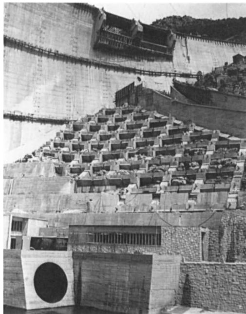
Fig. 8.10 View of the left abutment of the Grančarevo Dam with the field of large capacity rock anchors
