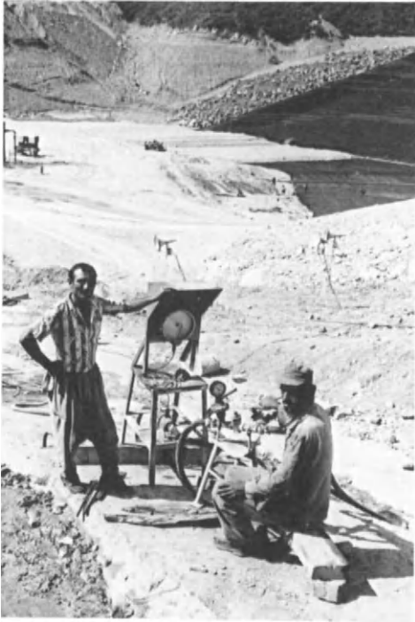
Fig. 6.40 Aslantas Dam, concrete slab in the foundation trench and grouting standpipe
