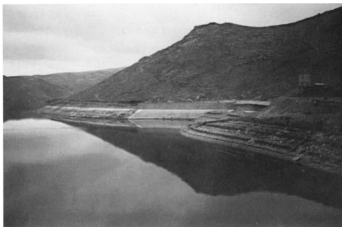
Fig. 6.25 Left shore of the Keban reservoir lined with concrete slabs
