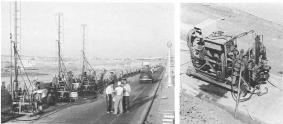
Fig. 5.2 Series of rotary rigs for the drilling of grout curtain through granite masonry at Aswan Dam (Egypt) and Diamec 250 rotary drill
