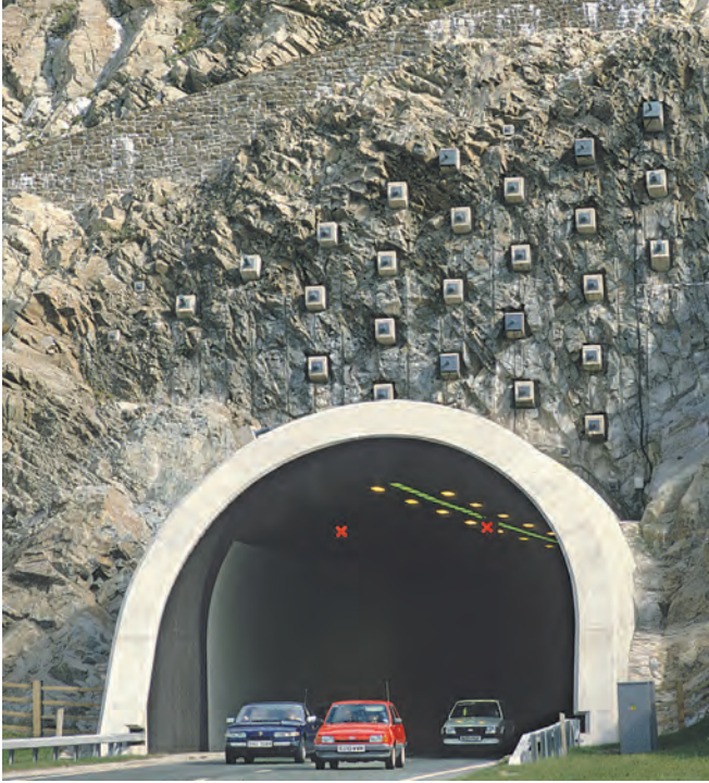
[above] The Pen y Clip Tunnel required massive steel arches for roof support through zones of fractured and deeply weathered rock. [left] The Penmaenbach Tunnel has rock anchors in the exposed face above the portal to prevent fractures opening by stress relief. [right] Parts of the Rhualt cutting had individual designs of anchors, rock bolts and dental masonry in dipping and faulted greywackes.
