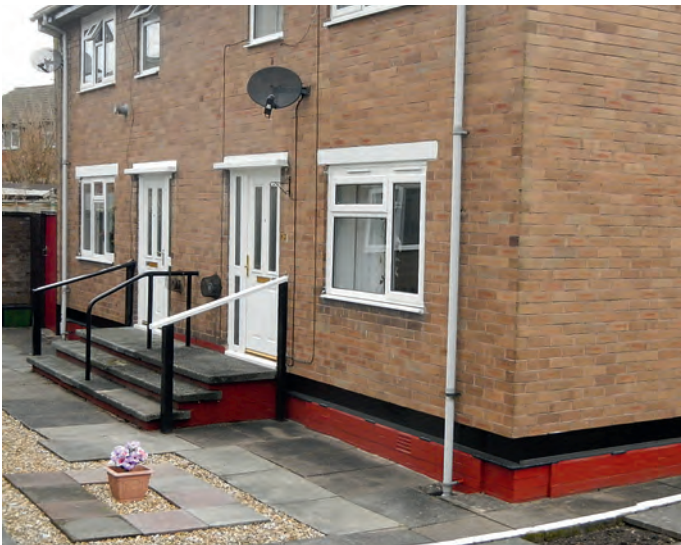
Houses on a black steel frame that can be jacked up, on salt karst with slow subsidence exacerbated by brine pumping.
