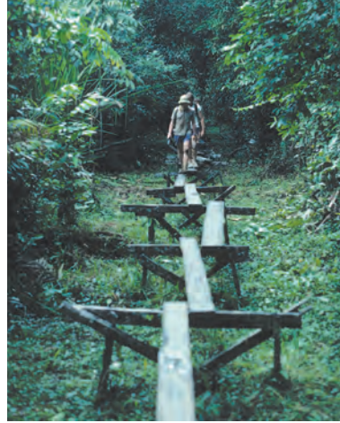
To link villages, forest dwellers use rot-proof ironwood to build raised walkways, because any heavy use turns a ground-level footpath into a mud quagmire.
