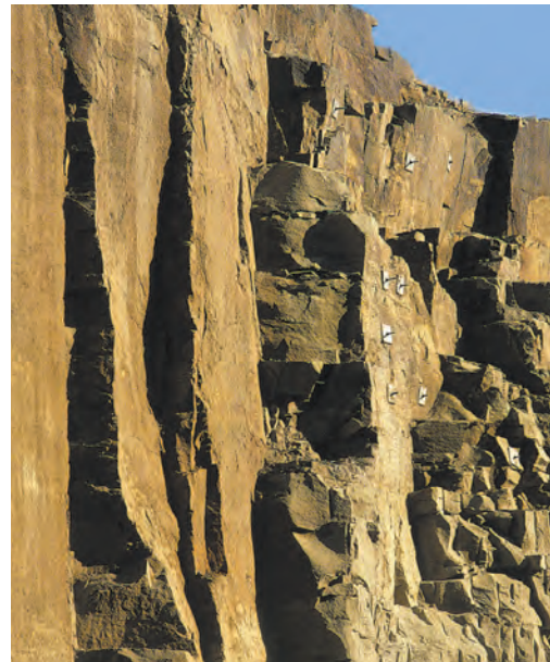
[left] A major unconformity with horizontal limestone above steeply dipping greywacke. [right] Vertical joints in massive sandstone, with rockbolts placed to keep the rock tight, dry and stable in a road cutting.
