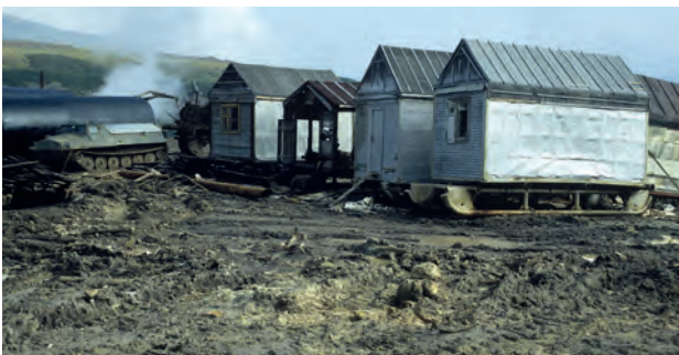
This house subsided when its own heat loss thawed the ground ice within unstable clay-rich alluvium.
