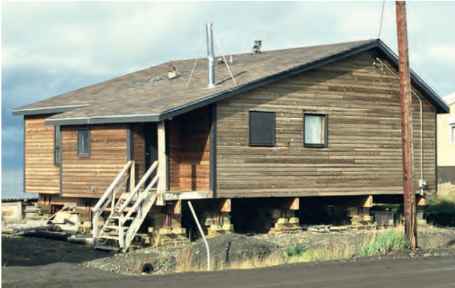
Enabling cold winter air to circulate freely beneath warm buildings ensures conservation of the permafrost; [left] house on wooden blocks on a gravel pad; [right] company building elevated on piles founded in ground ice.
