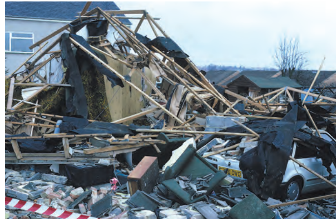
[above] Poor quarry after-use; this bungalow was destroyed by methane that filled it and exploded after flowing up-dip through a porous sandstone from a nearby quarry, which had been filled with rubbish and then sealed beneath a clay cap.
