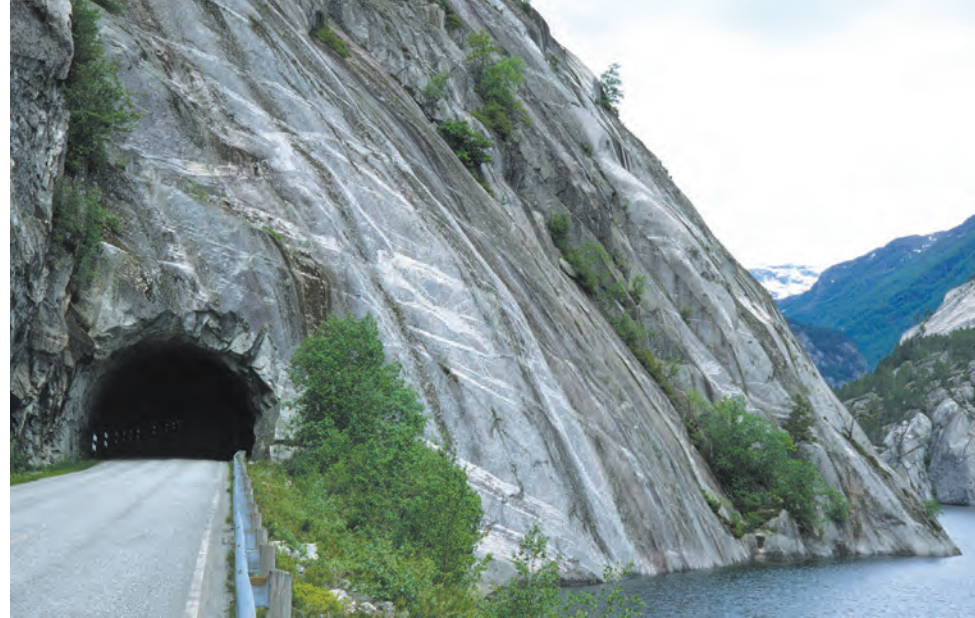
A steep mountain face is formed in structurally complex metamorphic gneiss with dipping banding and foliation, but the rock is strong enough to require no support within the road tunnel, mainly because it has a very low density of fractures.
