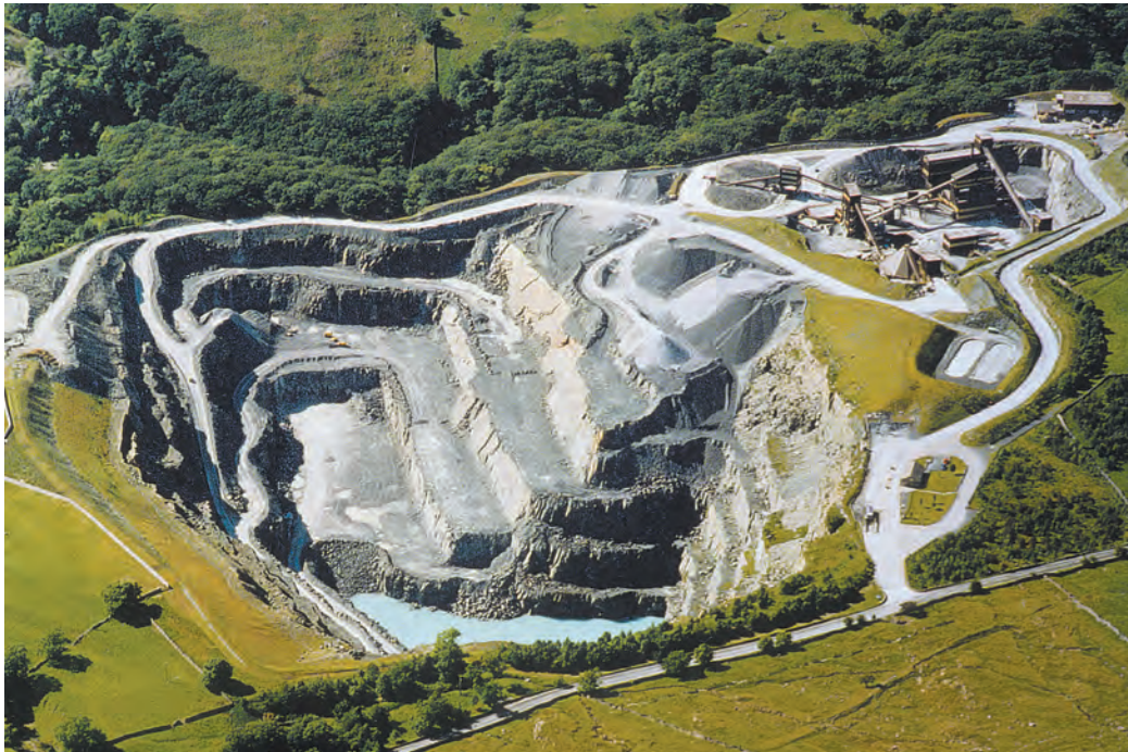
A small quarry works high-quality roadstone aggregate from steeply dipping greywacke. The site is constrained by a river on the far side, by the road in the foreground, and by adjacent slates left and right, with the crushing plant and stockpiles on slate to the right.
