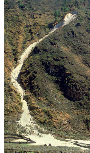
[above left] Large failure of deeply weathered rock with a debris slide that undermined a hillside road.
