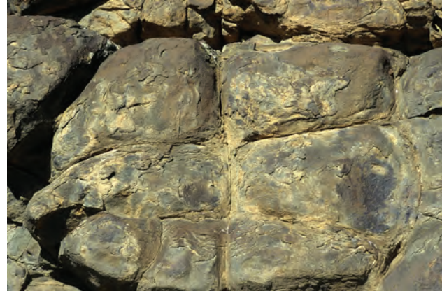
Chemical weathering of a dolerite with production of weak clay minerals first along the open joints 0.5m apart.
