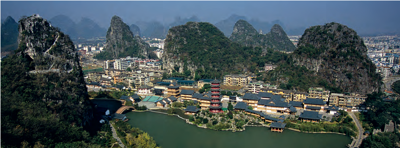
Buildings and infrastructure on the alluvial flats between the towers in karst of class kV may require foundations down to stable underlying bedrock or risk failure by development of new subsidence sinkholes within the alluvium.
