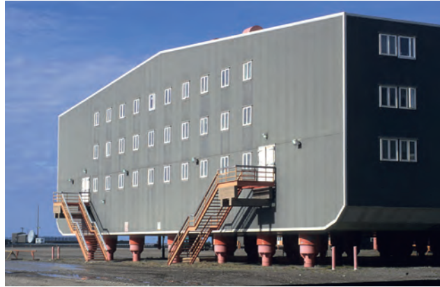
Enabling cold winter air to circulate freely beneath warm buildings ensures conservation of the permafrost; [left] house on wooden blocks on a gravel pad; [right] company building elevated on piles founded in ground ice.
