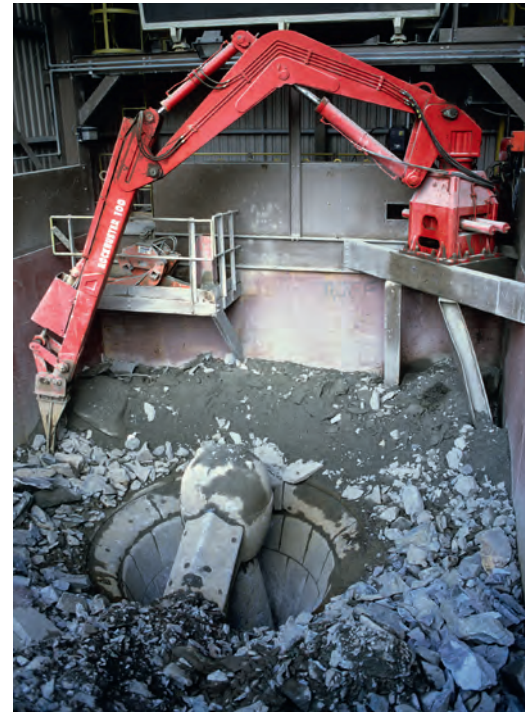
[right] The primary cone crusher at the same roadstone quarry, with its boom-mounted hammer to reduce any oversize quarry-run blocks.
