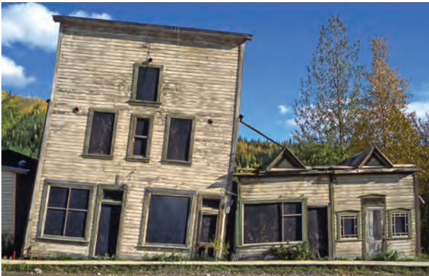
This house subsided when its own heat loss thawed the ground ice within unstable clay-rich alluvium.
