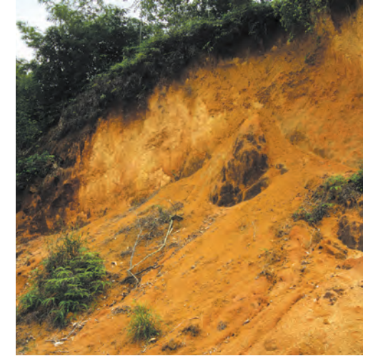
A thick, red, residual, kaolinitic soil of weathering grade V, which is the remains of a granite in a tropical environment.
