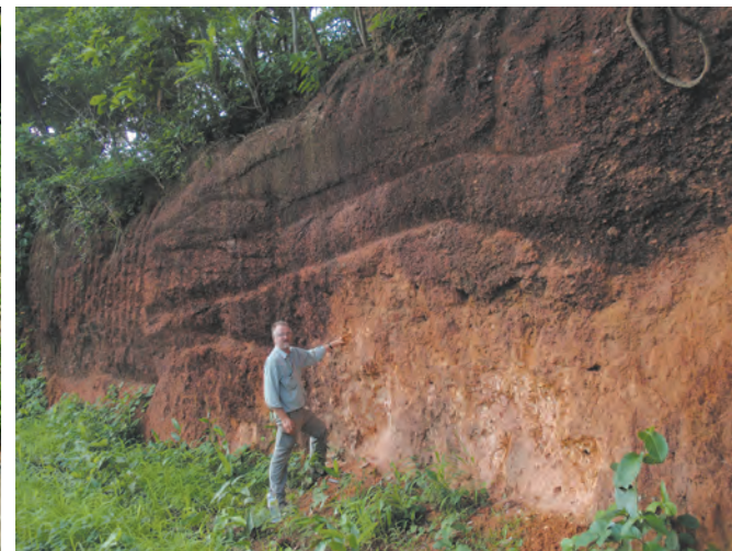
A cut face exposes completely weathered granite beneath a thick layer of residual soil that is largely ferricrete and therefore more resistant than the rock beneath.
