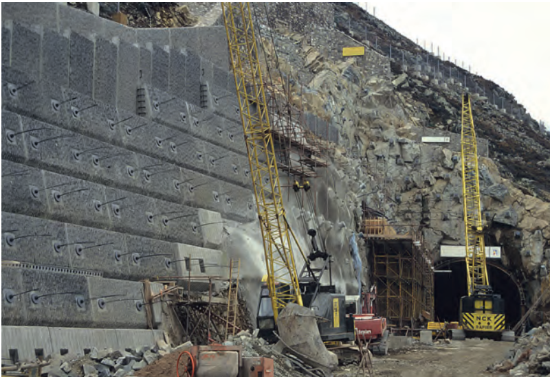
[left] Approaches to the Pen y Clip Tunnel have steep cut faces, where the unstable nature of the strong but densely fractured rock required continuous support by top-down construction of rows of anchored concrete panels.
