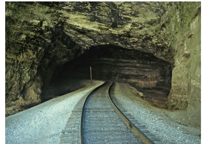
A rare benefit of mature cavernous karst in strong limestone, where a railway could be constructed inside a large cave in order to pass right through a high limestone ridge.
