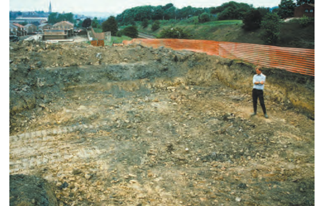
[upper right] A back-filled mine shaft 3 metres in diameter, recognisable by the darker fill where colliery waste about a metre deep had been stripped from the site, after the shaft was located by trenching through the cover across the area where it was suspected to lie.
