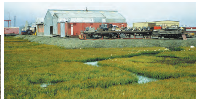
Summer canals over thawed ice wedges, beside a gravel pad that conserves the permafrost beneath the buildings.
