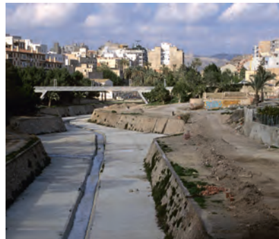
[below centre] Engineered channel through a town, designed to carry frequent floods from the adjacent mountains; normal flow is just in the central gully.
