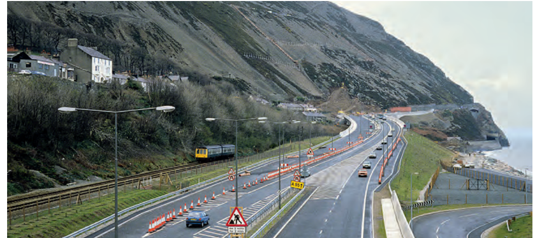
Parts of the coastal strip were an undercliff formed by the toes of landslides, and one area was stabilised by placing the road immediately behind a massive sea wall that was sufficiently massive to form an anchor weight over the rising part of the slip surface.
