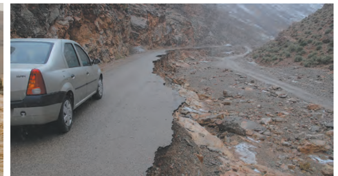
Desert road conditions: [from left] transverse corrugations on sand; flash flood through a desert town; flood erosion of a road embankment along a wadi, and a new track up its floor.
