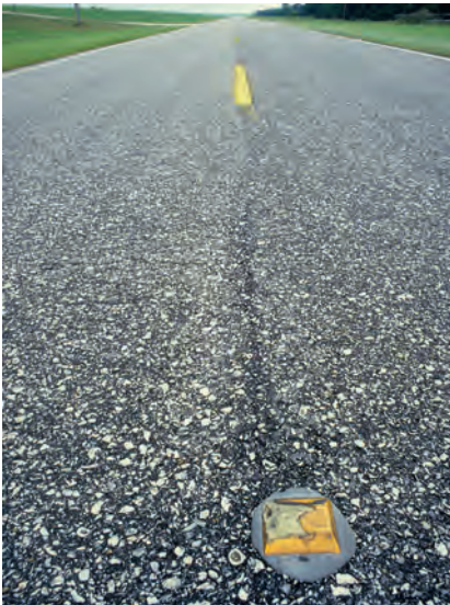
Dredged marine shells used as road aggregate; not widely acceptable as the calcite shells polish too easily and offer little skid-resistance.
