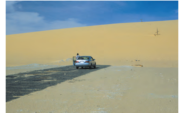
[left] Barchans are small sand dunes that migrate a few metres per year, here from right to left, due to wind from a single direction in Zone III. [right] The side of a single large barchan that has swept over a road, necessitating its re-routing.
