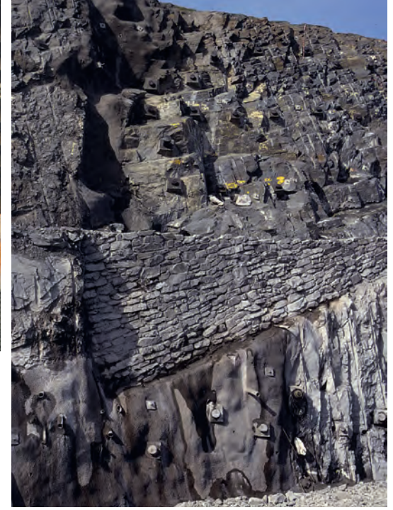
[above] The Pen y Clip Tunnel required massive steel arches for roof support through zones of fractured and deeply weathered rock. [left] The Penmaenbach Tunnel has rock anchors in the exposed face above the portal to prevent fractures opening by stress relief. [right] Parts of the Rhualt cutting had individual designs of anchors, rock bolts and dental masonry in dipping and faulted greywackes.
