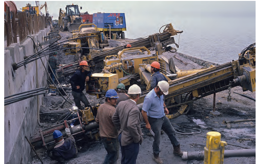
[left] Approaches to the Pen y Clip Tunnel have steep cut faces, where the unstable nature of the strong but densely fractured rock required continuous support by top-down construction of rows of anchored concrete panels.
