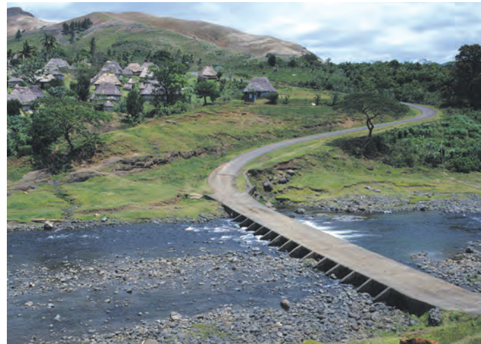
An "Irish crossing", or a flat bridge, across a flood-prone river floor in low-flow conditions; it was built with no parapets so that it causes minimal encroachment into the channel and frequent floods can pass over it with no damage to its structure.
