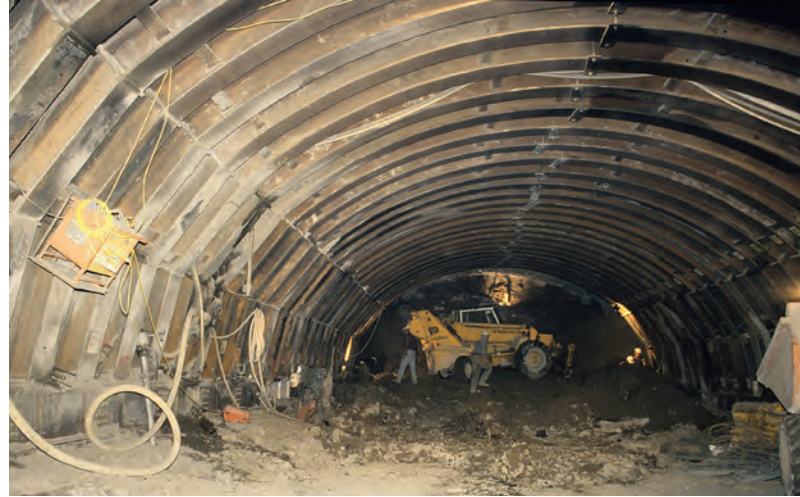
[above] The Pen y Clip Tunnel required massive steel arches for roof support through zones of fractured and deeply weathered rock. [left] The Penmaenbach Tunnel has rock anchors in the exposed face above the portal to prevent fractures opening by stress relief. [right] Parts of the Rhualt cutting had individual designs of anchors, rock bolts and dental masonry in dipping and faulted greywackes.
