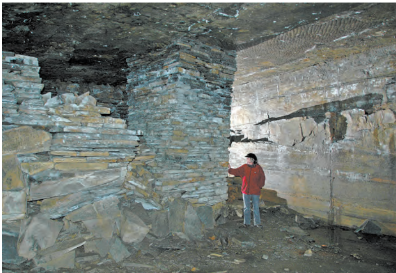
[below] Horizontal flagstone, sandstone that breaks into thin flags, in an old mine, with a roof support pillar made of waste flagstones.
