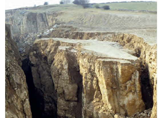
This large segment of wallrock subsided into an abandoned vein mine, which has since been backfilled to prevent wider ground failure.
