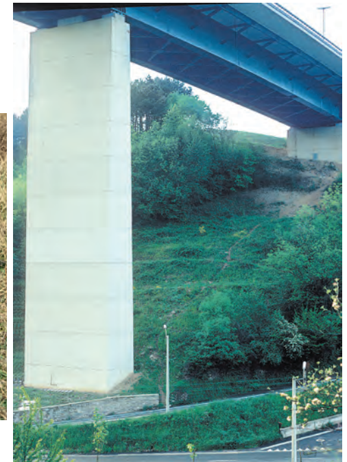
[below right] Viaduct pier that was relocated after an unpredicted cave (now beneath the grassy slope) was exposed only during excavation for the footing because it had been missed by all the investigation boreholes in karst of class kII.
