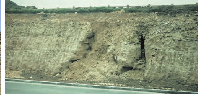
A camber fold over soft clay has open gullies in limestone that is sliding towards an adjacent valley off to the right.
