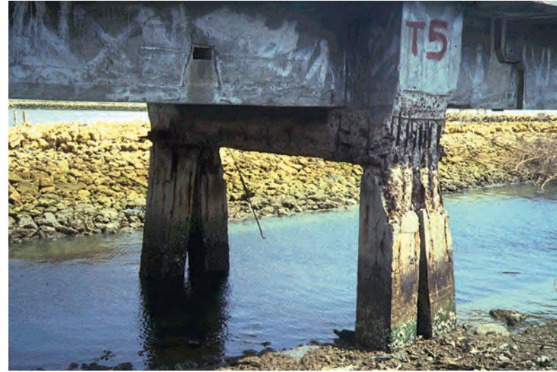
Chemical attack on poor concrete, and subsequent corrosion of its steel reinforcement bars, at the inter-tidal level of a marine structure.
