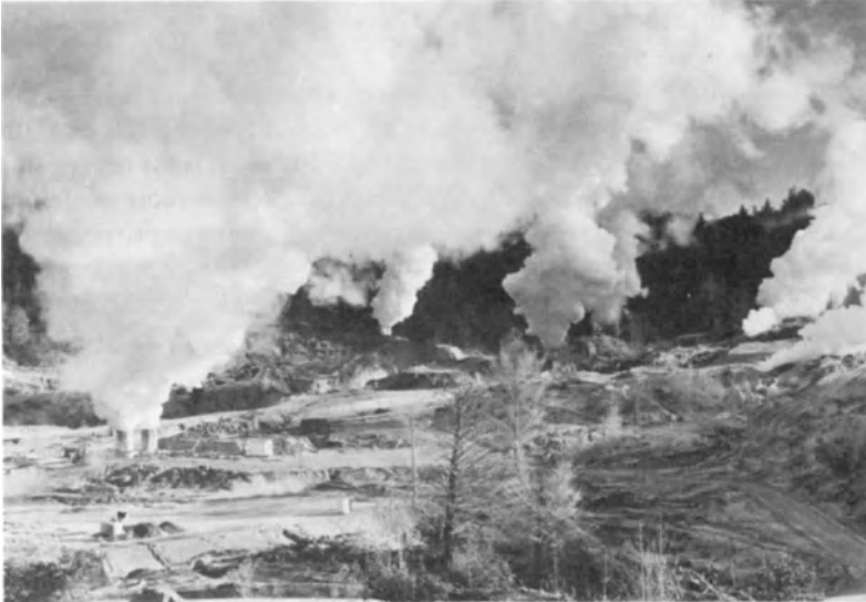
FIG. 4.28. Vertical twin-tower silencers forming part of the standard equipment at each wellhead (Wairakei). Reproduced by courtesy of The High Commissioner for New Zealand, London.
