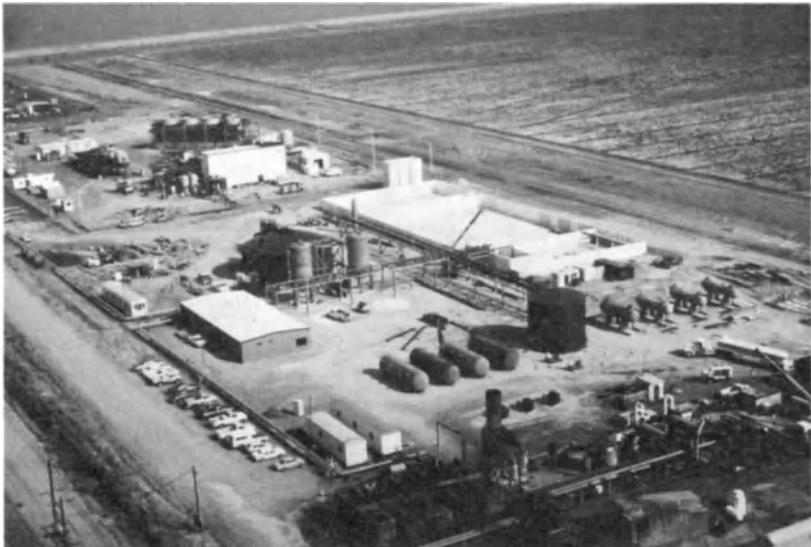
FIG. 4.5. Brawley, California, USA: 10-MW single-flash geothermal demonstration facility in operation. This was dismantled after the successful demonstration. Reproduced by courtesy of the Southern California Edison Company, California, USA.
