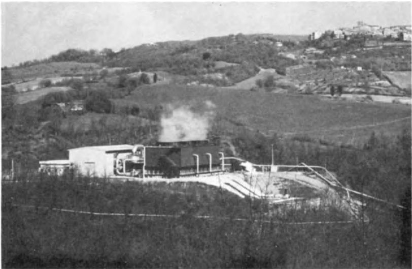
FIG. 4.13. Le Rancia power station, Travale-Radicondoli.
