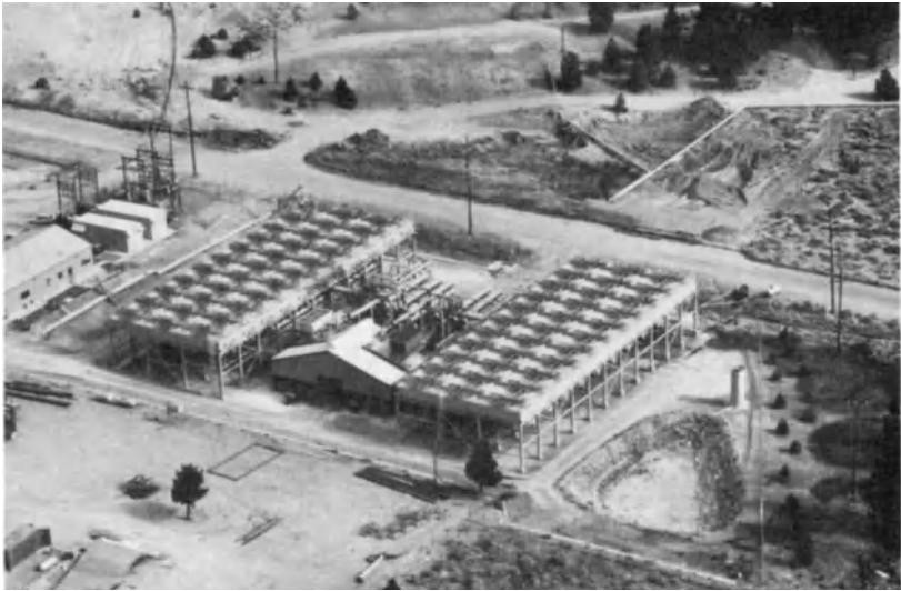
FIG. 4.4. Mammoth Lakes, California, USA: 7-MW binary-cycle geothermal project designed and operated by the Ben Holt company. Reproduced by courtesy of the Southern California Edison Company, California, USA.
