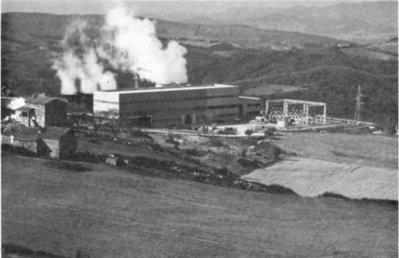
FIG. 4.12. San Martino power station, Larderello.
