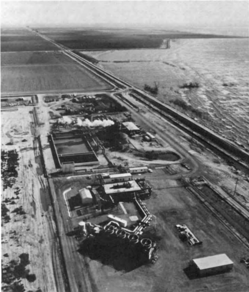
FIG. 2.9. The Salton Sea, California, USA. Geothermoelectric power plant on the shore of the Salton Sea in southern California taps hot brine which is highly corrosive. Most of it is re-injected, but some is removed by trucks. Reproduced by courtesy of the Southern California Edison Company, California, USA.
