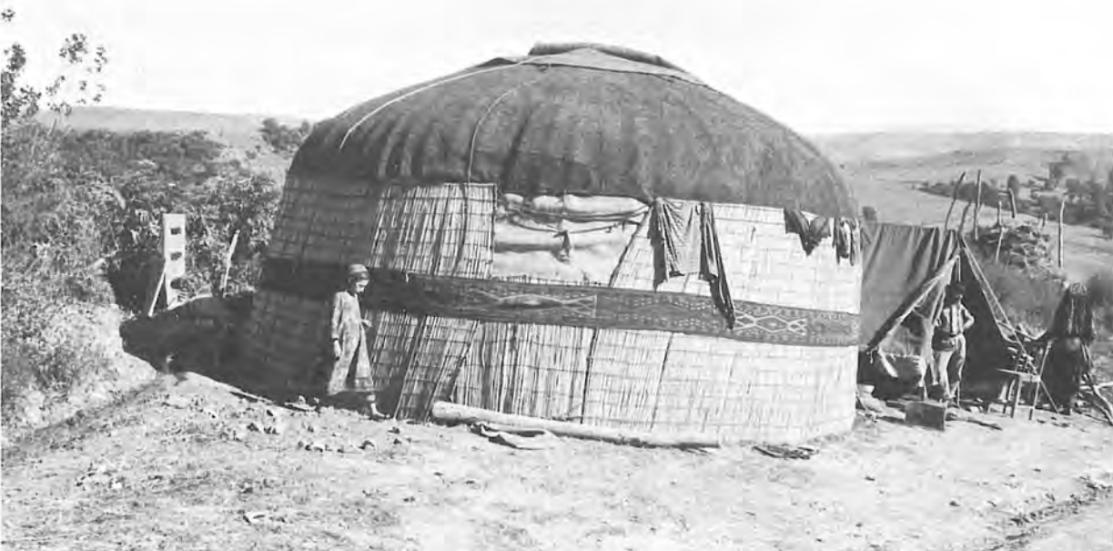
Plate 3. Turkoman yurt in northeastern Iran after the destructive earthquake of 30 July 1970.
