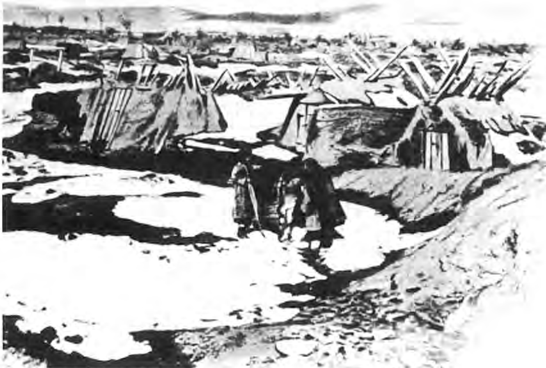
Plate 27. A-shaped shelters put up in Quchan after the earthquakes of 1893 and 1895. Other views of this type of construction are shown in Huntington (1905: 236) and MacGregor (1879: 85).
