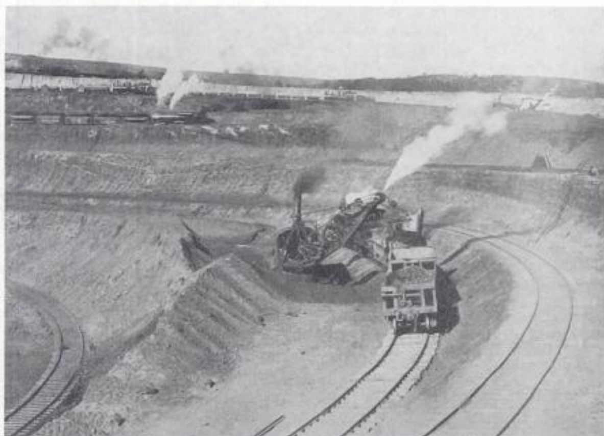
Figure 1.10. Steam shovel mining of ore (Van Barneveld, 1913).
